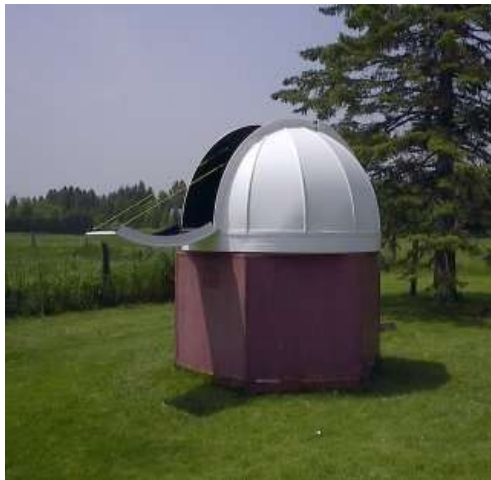
Figure 8 – Draw Bridge Shutter Design
